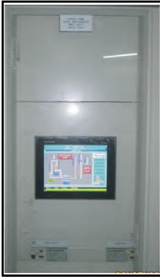
Figure 9: AWLS PLC Control Panel
