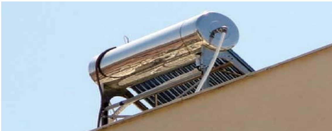
Figure 6: A solar water heater on the roof of the building of a Jordanian private Hospital
