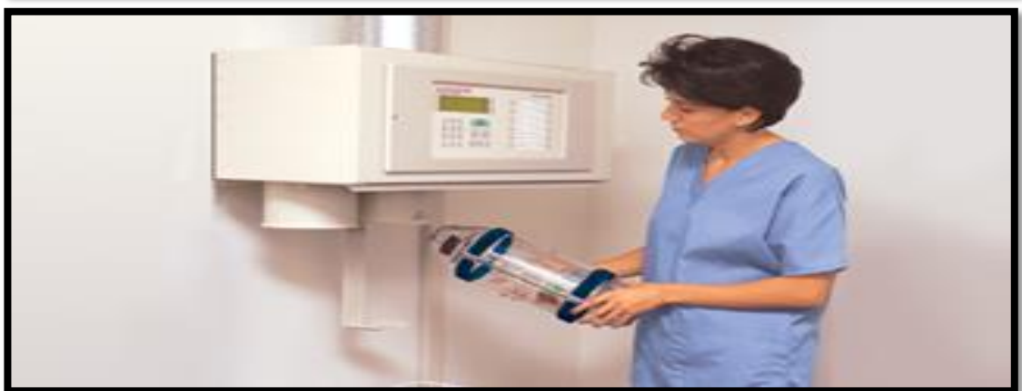
FIGURE: 5.16 PNEUMATIC TUBE STATION – WALL MOUNTED AND COUNTER TOP SHOWING CARRIER CONTAINERS
